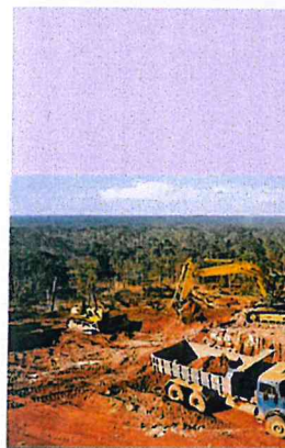
Iron Ore Mines
